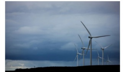
Vestas wind turbines in Germany. Image by: Vestas Wind Systems A/S.
